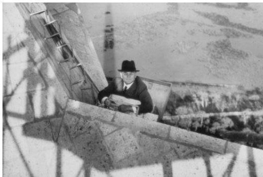
Brother Alfred C Finn, Architect of the San Jacinto monument, pictured above inspecting the construction of the monument.
